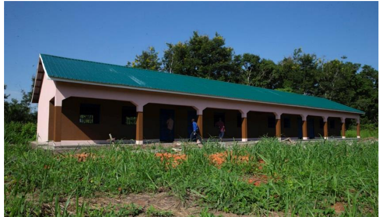
The new classroom block in Bazumburu constructed by UNMISS.
