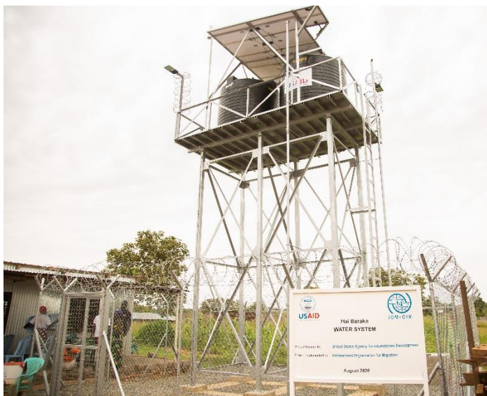
The hybrid solar system water Yard in Hai Baraka. Photo Credit IOM
